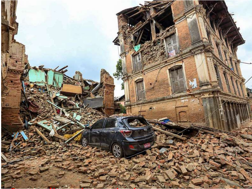
Damages of houses due to earthquake Source:Nepali Sansar
