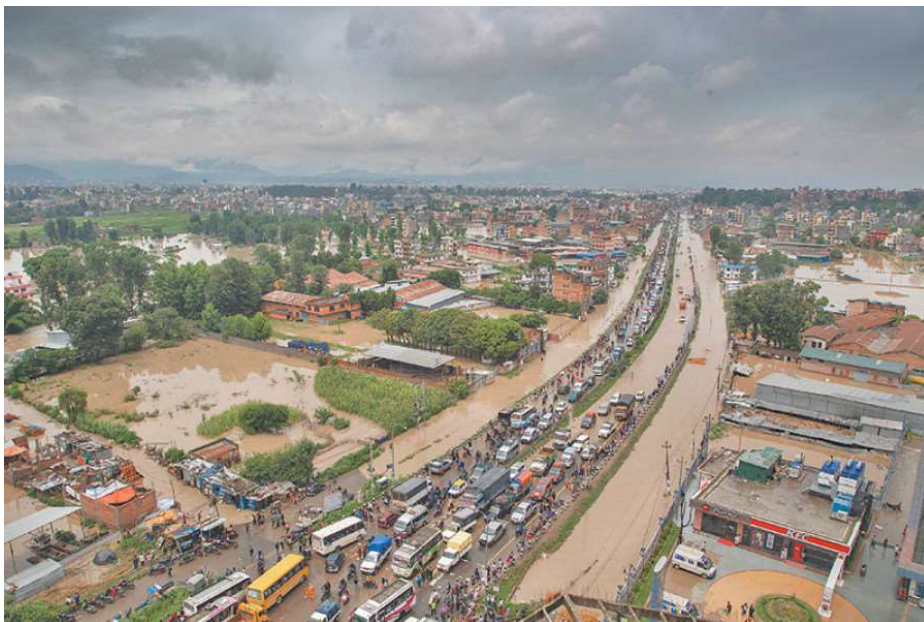
Road and traffic after flood in Bhaktapur Source: The Kathmandu Post
