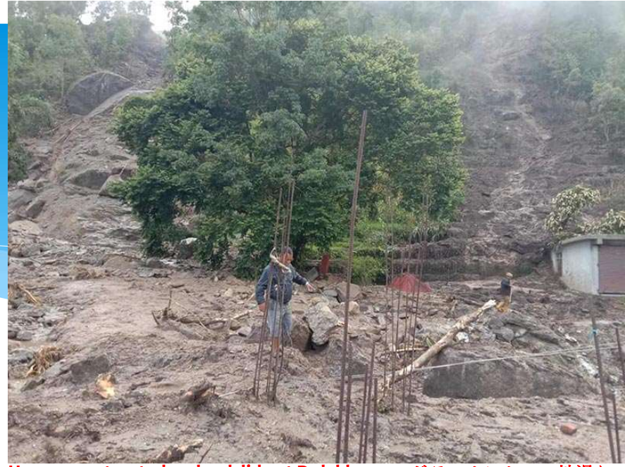
House constructed on landslide at Dolakha Source: The Himalaya Times
