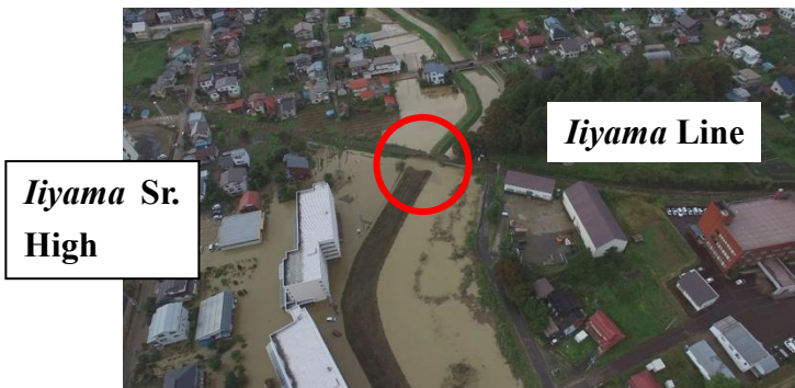
Fig. 7 Site of Sara-gawa Collapse (provided by iNet)
