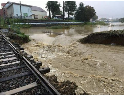
Fig. 5 Collapse of the Sara-gawa River (6:00AM, Oct. 13 th )
