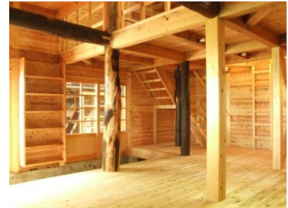
Small mountain hut reconstructed by T. Tsuchimoto and his colleague integrating the old and the new after detailed survey.
