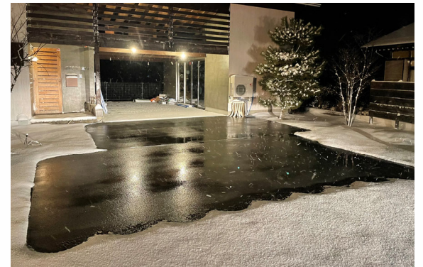
Hybrid snow melting pavement: eco-friendly snow-melting pavement that combines concrete pavement with synthetic graphite with high thermal conductivity and a heat pump.
