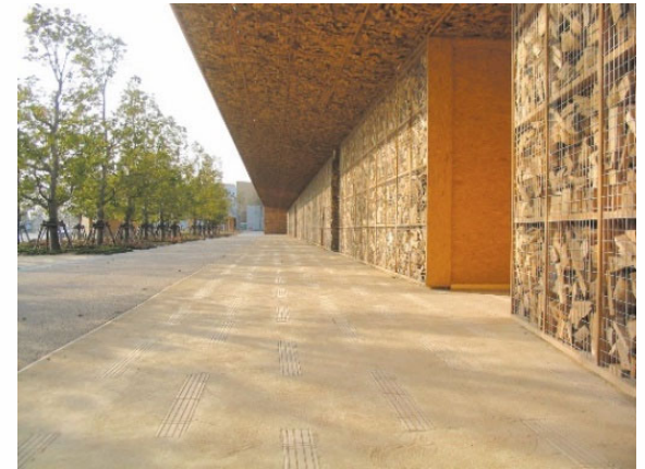
Soil pavement: eco-friendly and human-friendly pedestrian pavement.
