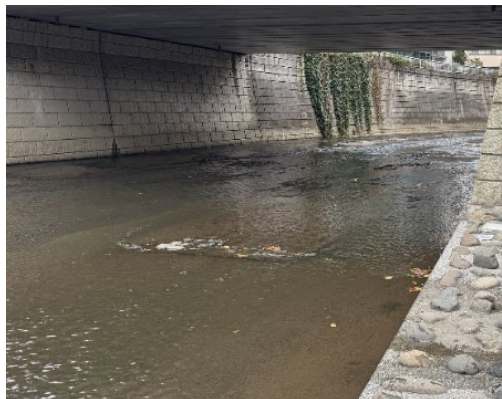
Fig.2 Concrete riverbed at Kanda river.
