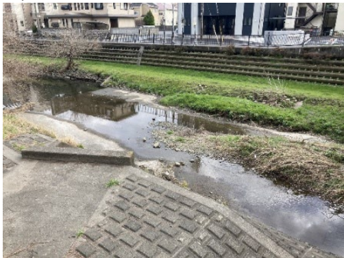
Fig.1 Concrete riverbed at Nogawa river.
