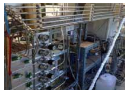
A power-generating device that uses a solid oxide fuel cell
