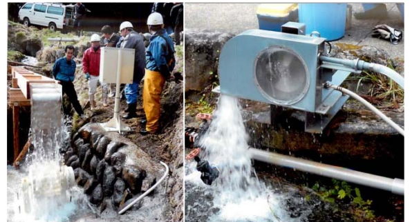
Waterfall type turbine ( left ) and Jet type turbine (right) Each electric power is used for an electrified fence and a satellite mobile phone.
