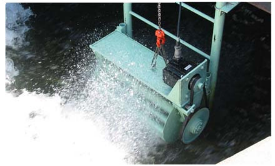
Photo of opened undershot type turbine. The electric power is used for lighting in a house.
