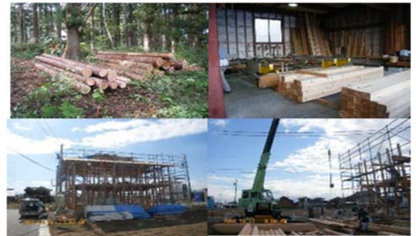
Process of lumber from log to house construction through sawing
