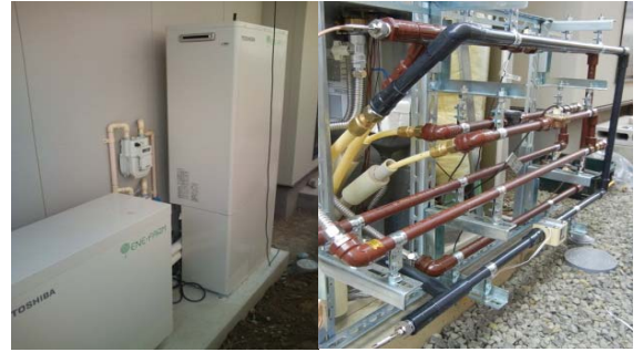
Residential fuel cell co-generation system which supplies electricity and hot water.
